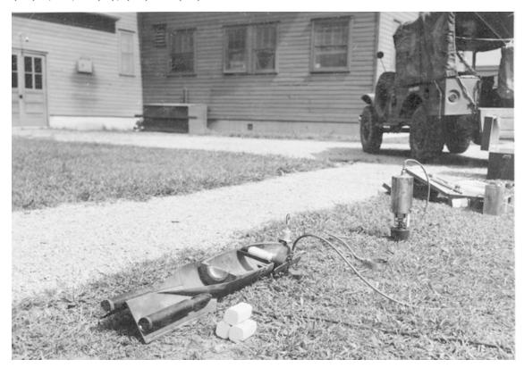
The building in the background was a barracks for the enlisted bomb disposal students. The truck in the background is the WC-51 3/4 ton 4x4 Dodge, part of the BD authorization. Also in the background, on the ground behind the steam boiler, is the T-17/M-1 Grease Gun Pump. It was used
