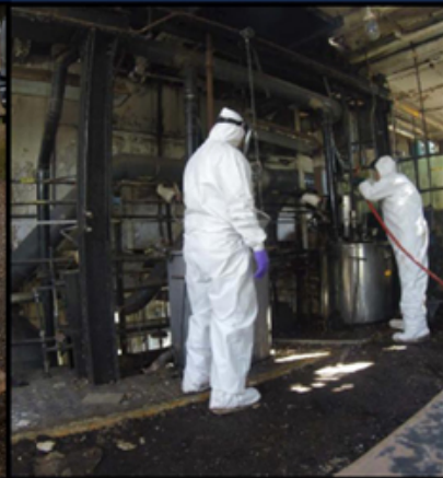
Building and Equipment Decontamination
