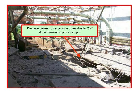
As far as we know, when the operating contractor laid away this building in the 1970s, he followed proper procedure by flushing the pipe. The flushing was intended to remove large quantities of explosives, but cannot guarantee complete removal of all explosives. The 3X designation means that dangerous quantities of explosives could still remain. In this case, they did remain.
