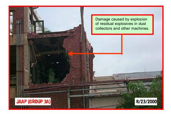
9. Joliet AAP. This explosion occurred during remote cutting of a decontaminated (3X) process water pipe.
