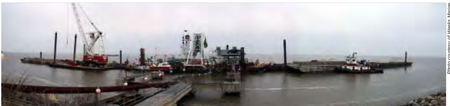
Dredged material from Baltimore Harbor Anchorages and Channels project is unloaded at the Hart-Miller Island pier.
