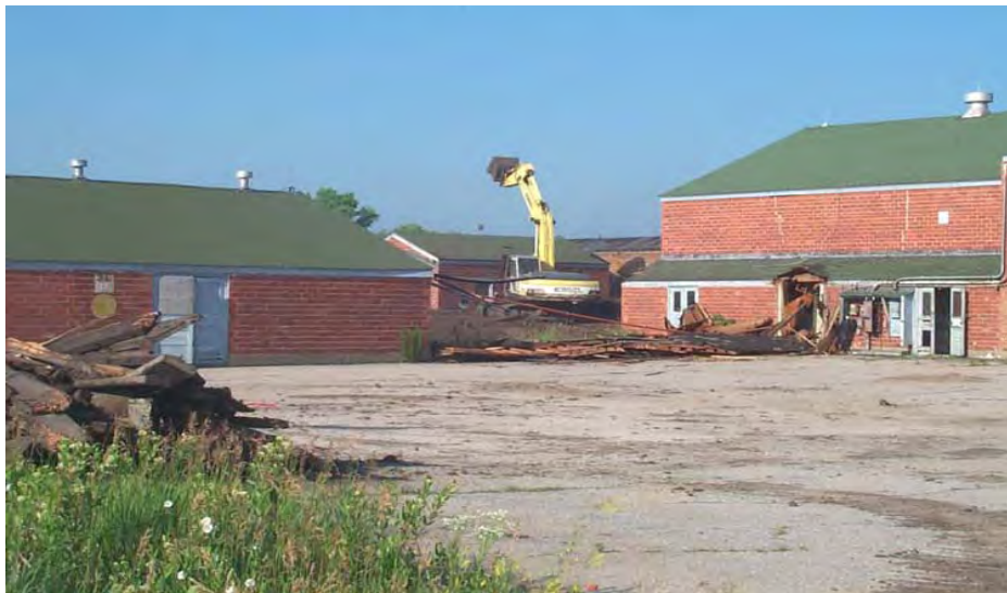
Building Remediation/Demolition Cornhusker AAP
