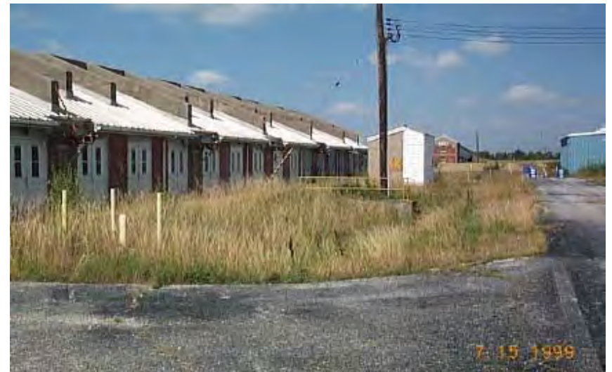
Building Remediation/Demolition Kansas AAP
