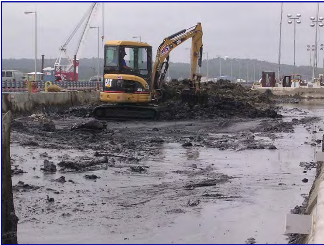
Dredge Spoils Screening Operation
