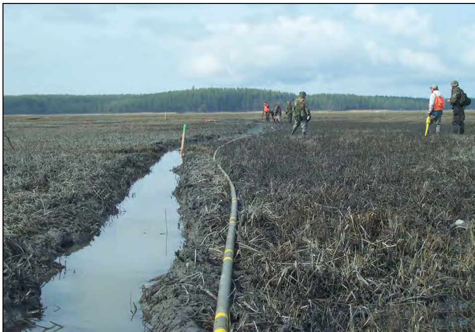
Figure 7. Laying out Bangalore torpedoes.
