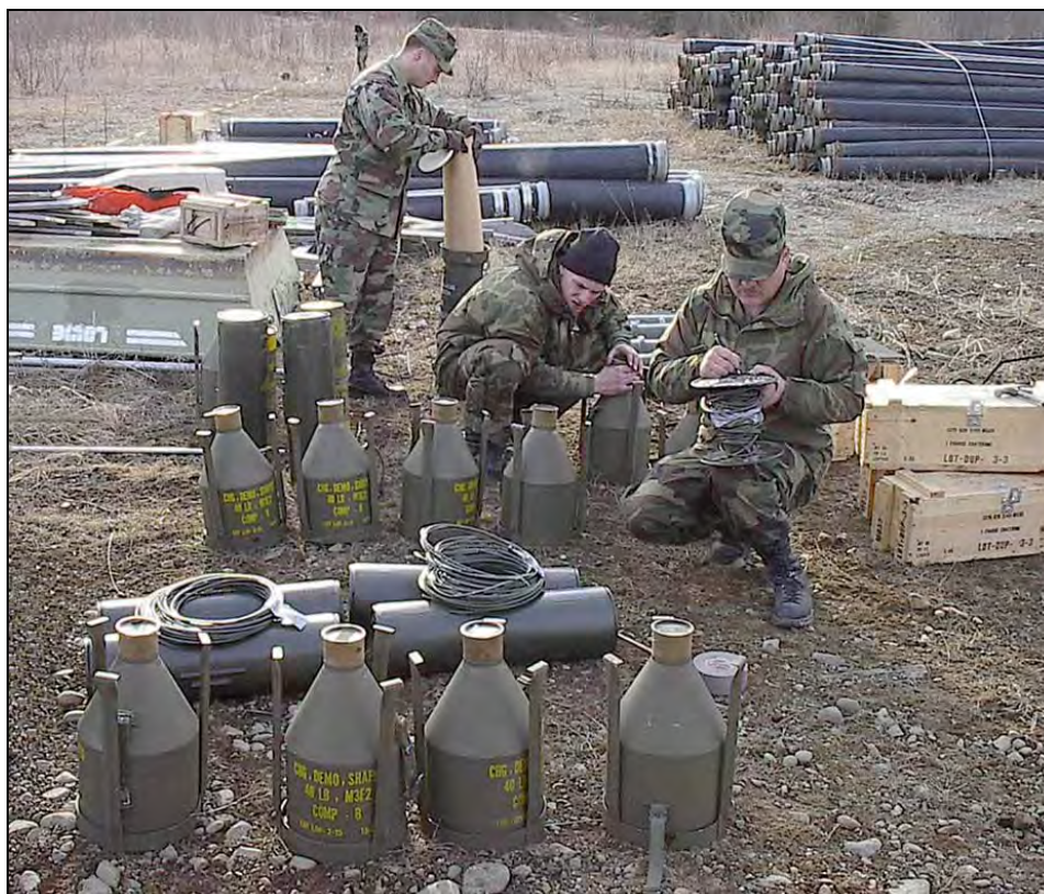
Figure 4. Preparation of shaped (foreground) and cratering charges.
