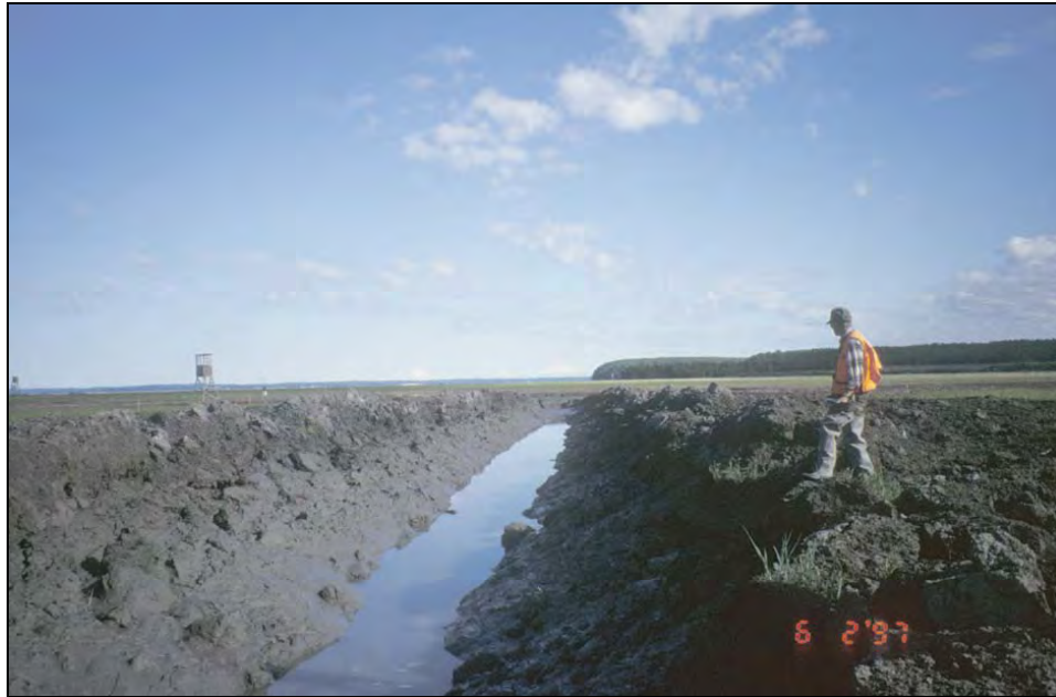
Figure 6. Drainage ditch at Pond 293 (cratering charges).
