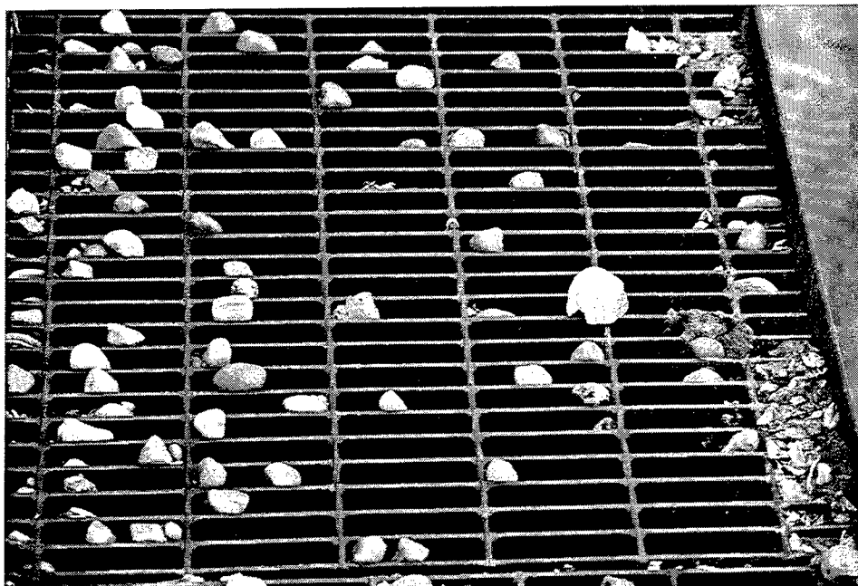
Figure 9. Blinded-off bar grate separation screens
