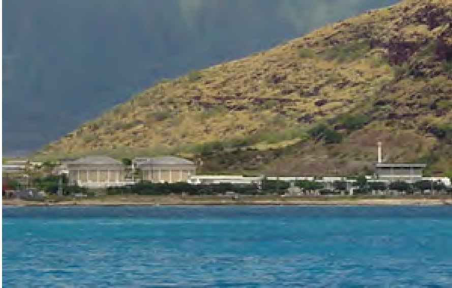
Figure 4. The Wai'anāe Wastewater Treatment Plant (WWTP) , Source: CZM Hawai'i
